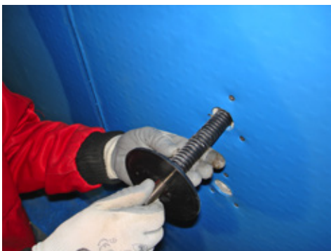
Figure 33: Carefully assembling (screwing) into the plastic resin.
