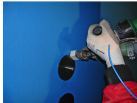
Figure 35: Extrusion welding of the mounted BA-anchor
