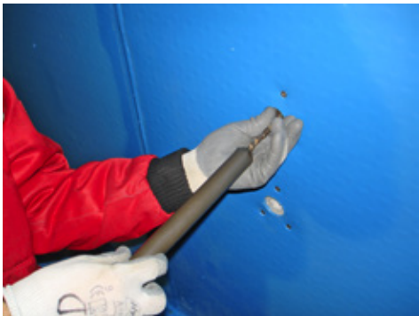
Figure 32: Assembling of the resin cartridge
