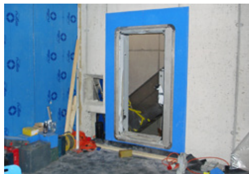
Figure 46: Assembled pressure tight door
