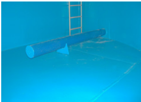
Figure 43: Pipe support with PE pipe
