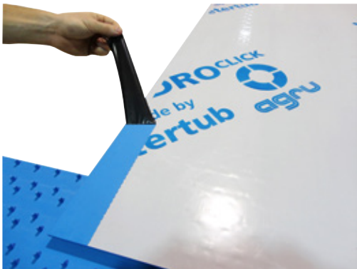
Figure 4: Removal of the protective film at the welding area
